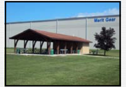
Hudson Street Shelter
